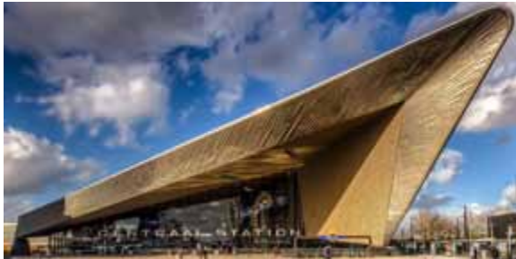
Figure 45 Rotterdam Central Station-Netherlands http://www.archdaily.com/
