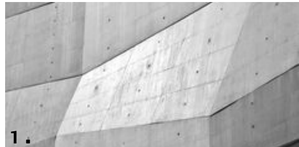
Figure 77 Station materials (continues on next page)
