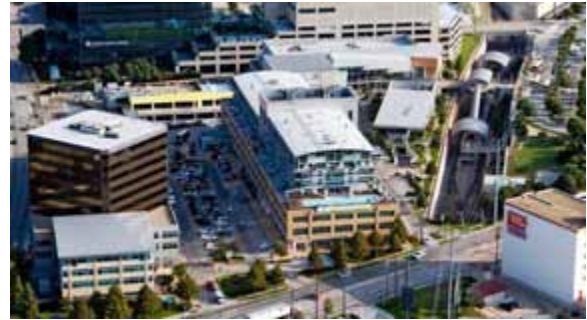
Figure 36 Mockingbird Station Aerial View http://dartdallas.dart.org/
