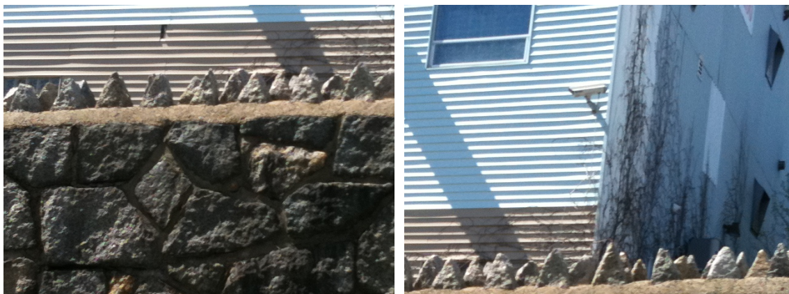
Figure 4.7: Stone Wall Scene (a) Left View, (b) Right View
