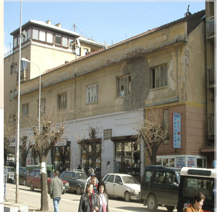
Fig.7.0. A view from a damaged façade of a joint dwelling in Pristina
