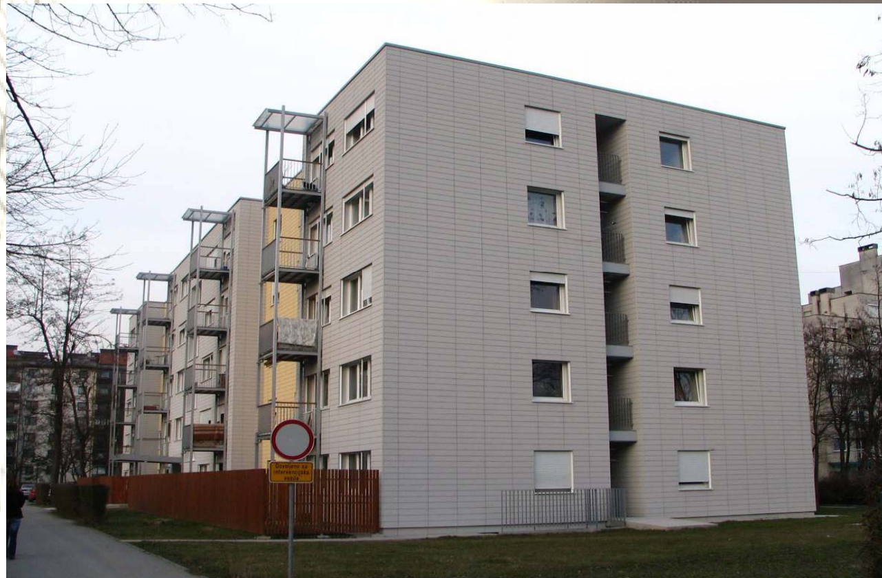
Fig 1.0.: Apartment building Hermana Potočnika 17 after renovation
