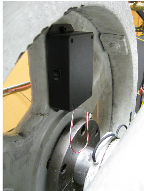
(b) Wireless accelerometer with transmitter box
