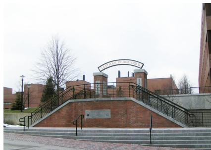
This campus site offers the use of multiple, adjacent staircases.
