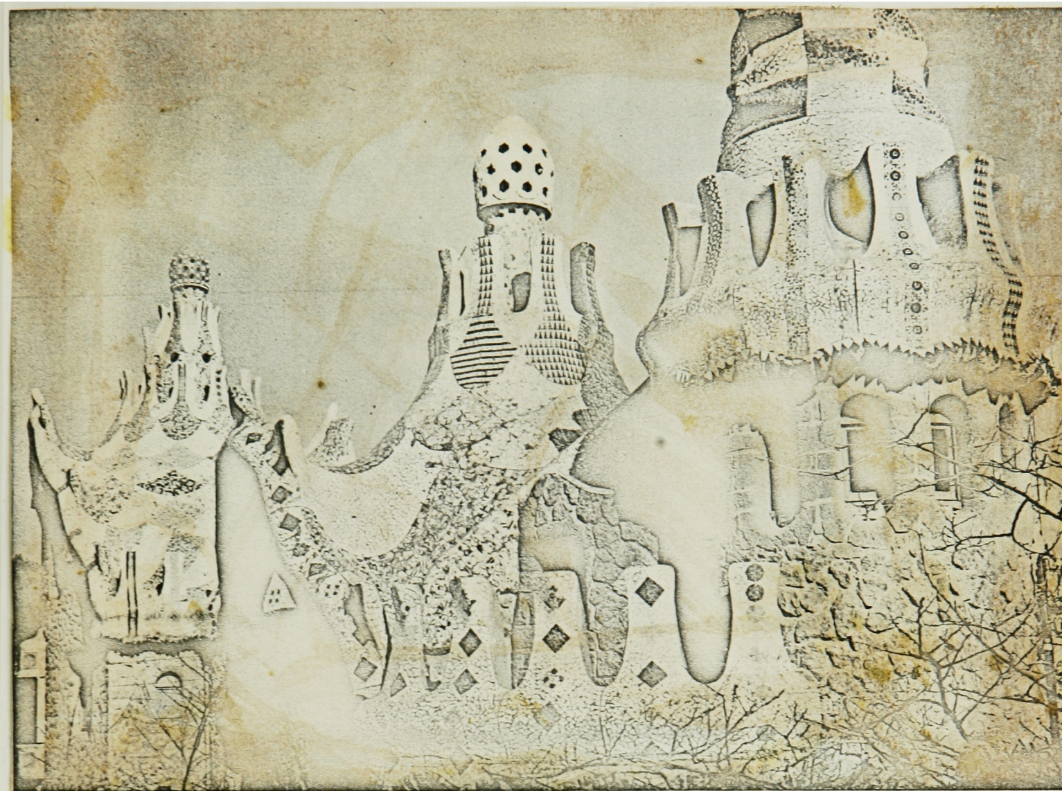
68. Roofs and crowning members of the two gate lodges of the Park Güell. The two perforated pinnacles are actually chimney pots.
