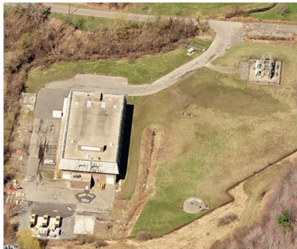
Figure 3.3: The pump station and transformer yard that bring wastewater to the Van Lare facility from Irondequoit.
