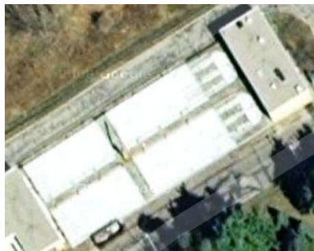
Figure 3.7: West side aeration tanks, which are covered because the air is added to the mixture through pipes at the bottom of the tank.
