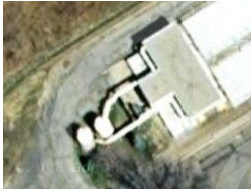
Figure 3.4: West side screening and grit removal building, which uses large moving screens to grab the objects and pull them out of the liquid and into a garbage bin, then spins the wastewater to cause grit to settle to the bottom.
