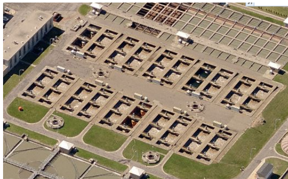
Figure 3.8: East side aeration tanks that vigorously stir the wastewater.
