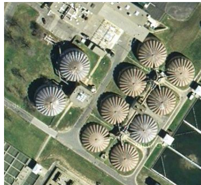
Figure 3.14: Evaporators or thickeners, these large structures are long term settling tanks for sludge.
