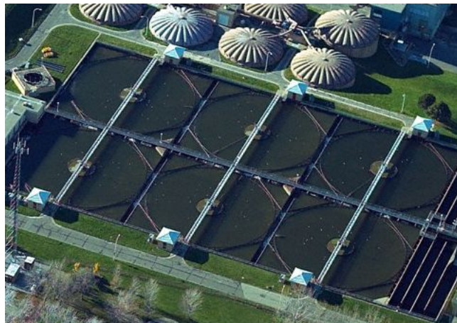
Figure 3.11: The six large secondary settling tanks.
