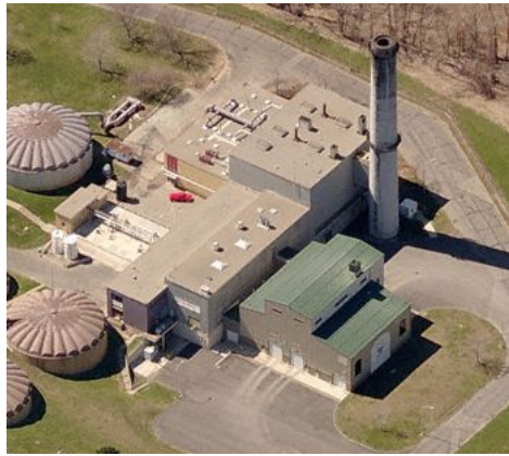
Figure 3.15: The group of buildings that deal with sludge treatment.
