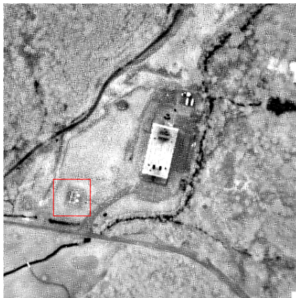
Figure 2.14: LWIR image of the Irondequoit pump house at the Van Lare facility and a transformer yard (outlined in red) that is directly related to the power usage of the building.
