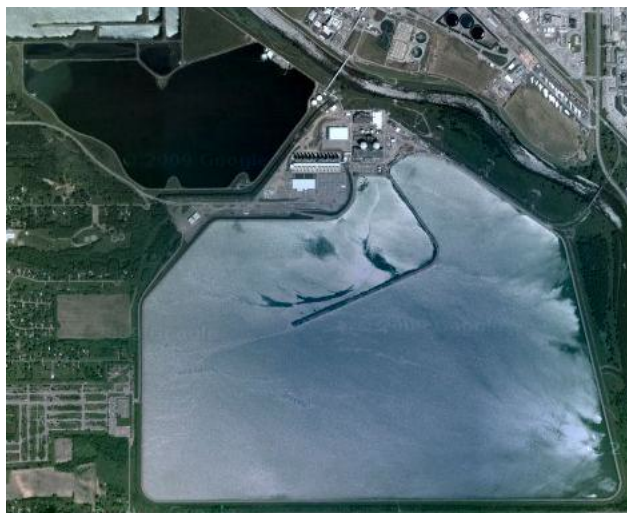
Figure 2.7: A relatively small facility with a giant cooling pond. The large electrical transformers give away that this is a power plant. Image courtesy of Google Earth.
