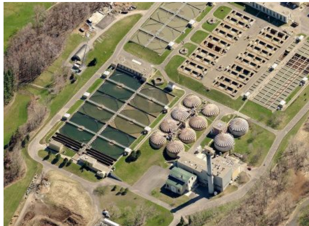
Figure 4.9: An image of the secondary settling tanks on day when the biological balance was not maintained perfectly and they ended up very cloudy. Image courtesy of Bing Maps.
