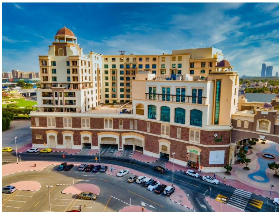
Figure 1. Oud Metha Plaza Building
