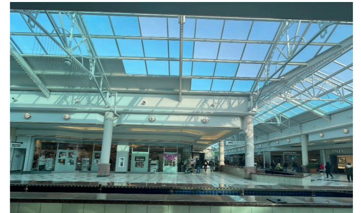
Figure 23: Existing Condition-Skylight, Photo by Qianyue Tu, Accessed 01 May, 2023.
