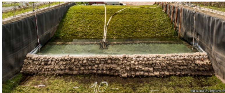
Fig 4. Sandbags dam be covered with a protruding plastic apron
