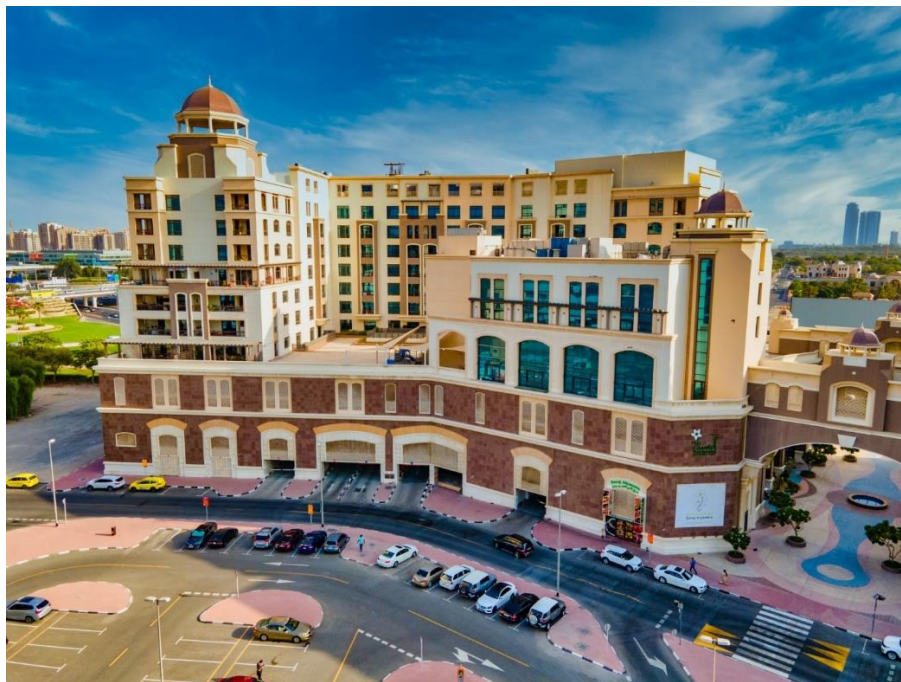
Figure 1. Oud Metha Plaza Building
