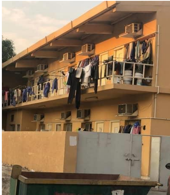
Figure 10: The phenomenon of spreading cloths in balconies
