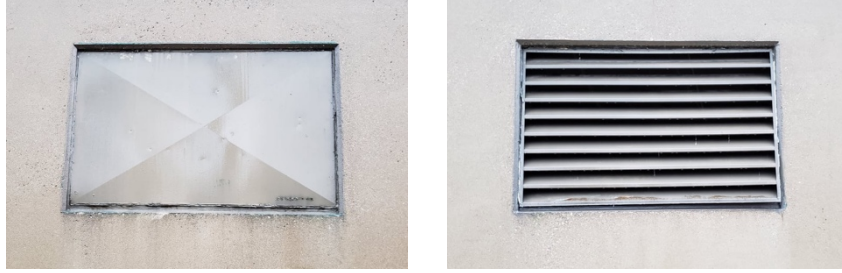
Figure 2: Found exterior panels – AMSCO (Erie, PA)
