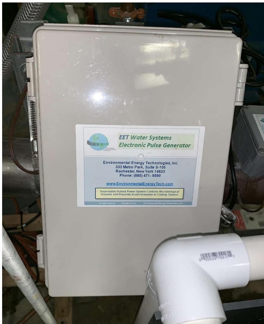
Figure 2: EPG developed by EET.
