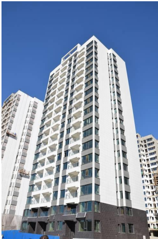
Figure 15 Building C15, Qinhuangdao, China (Source: https://wenku.baidu.com/view/8d773e0a77232f60ddcca17f.html )
