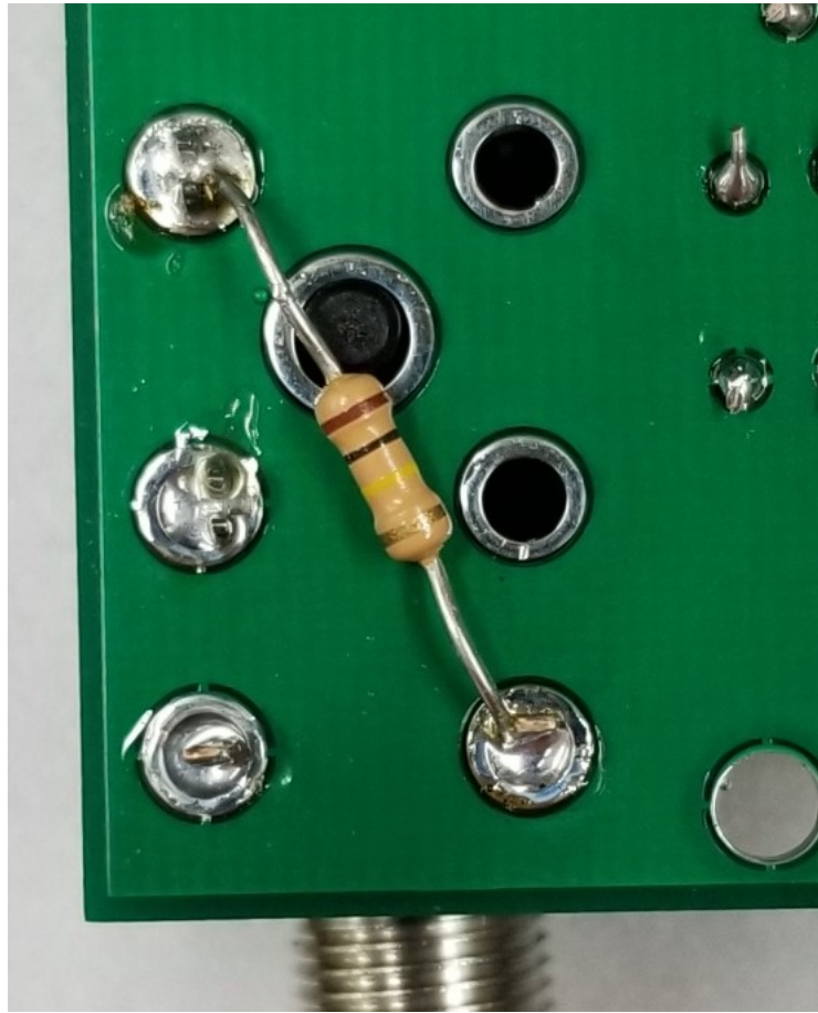
Figure 5.1: Fix to prevent large DC voltages at the output of the circuit upon power on.
