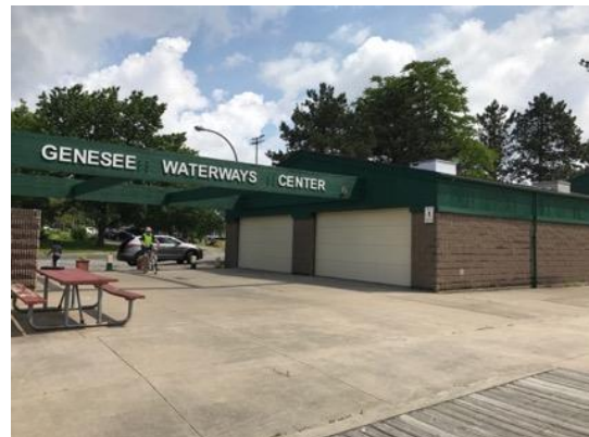
Figure 36: GWC Small Storage, source: author
