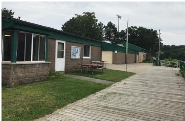
Figure 35: GWC South Elevation, source: author
