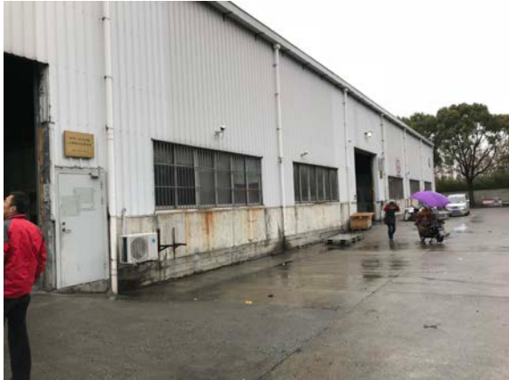
Figure 17 Exterior facade of Warehouse
