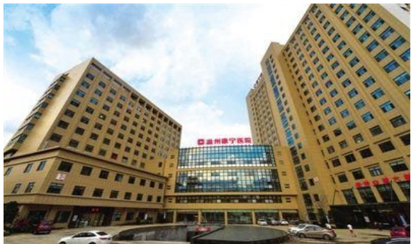
Figure 31 Wenzhou Kangning Hospital
