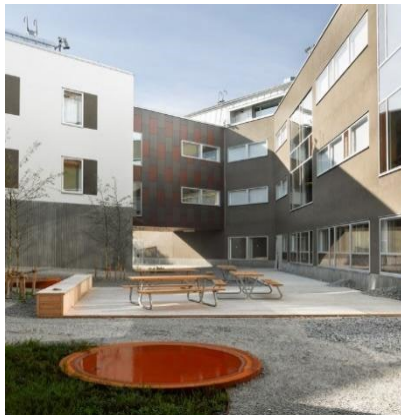
Figure 23 6-meter-high wall around the facility
