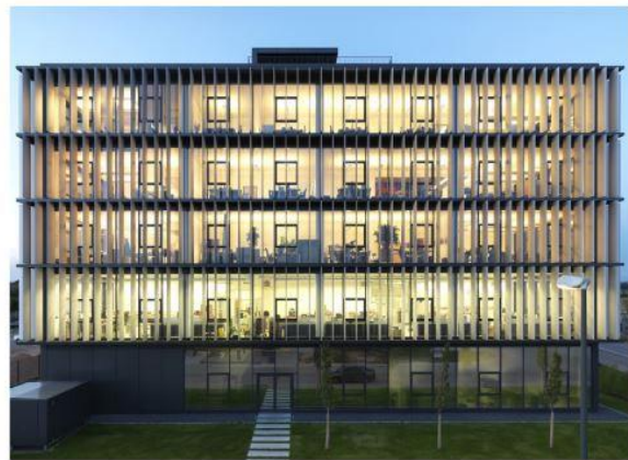
Figure 11. Silver Alucobond Louvers in Gaimersheim Germany Designed by Kandler-Bunje Architects + Engineers https://www.alucobondusa.com/blog/silver-alucobond-louvers-provide-innovative-daylighting-to-facade/#.WhZFYrpFxEY
