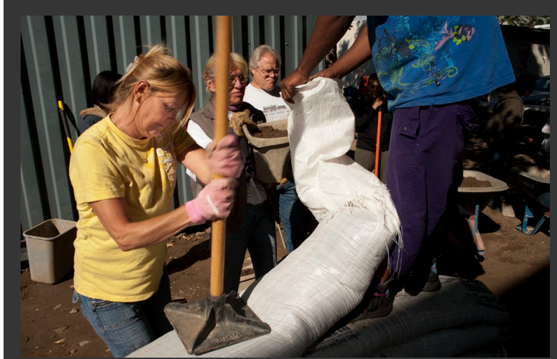
Earth is poured into bags and beaten flat to make the walls of the Eco-Dome structure.
