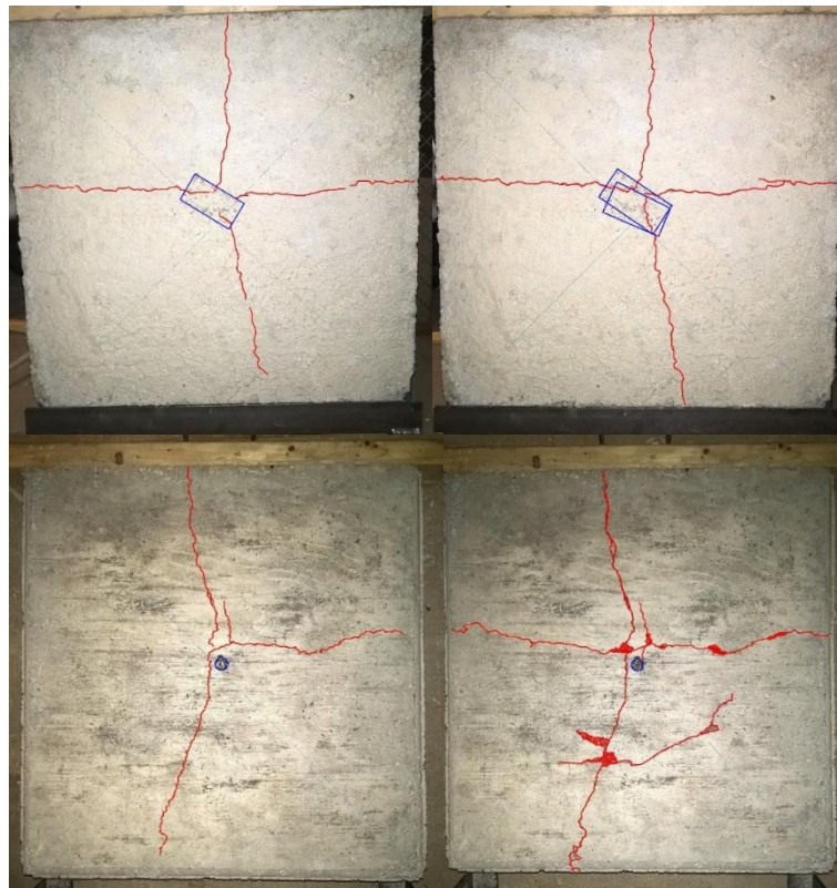
Figure 4.10. The front (top) and back (bottom) faces of the slab after impacts. Images on the left show impact 1, images on the right show impact 2. Formed cracks and areas of spalling are shown in red. Accelerometer location and wood projectile location are shown in blue.
