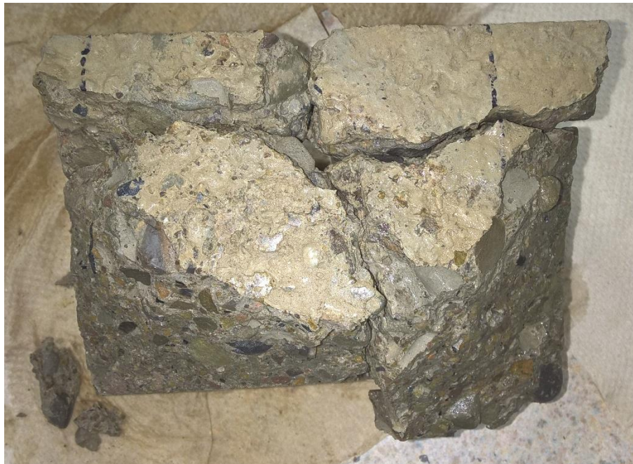
Figure 4.11. The cross section of the impact zone, showing a plug-like conical cracking pattern along the bottom of the sample. The cavity can be seen in the center of the sectioned block.
