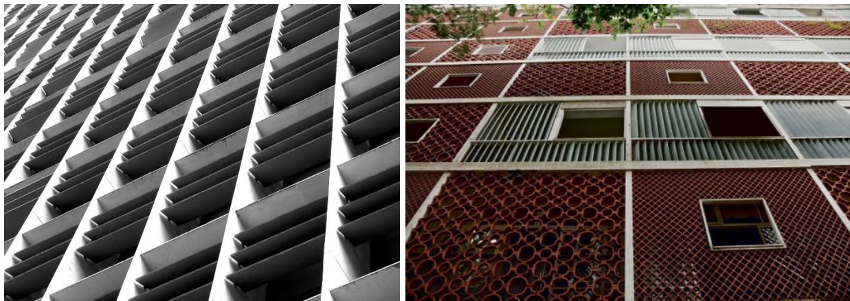
Figure 23 - Brise-soleil at the Ministry of Education and Heath (Lucio Costa)(left) and cobogós at the Bristol Building (Lucio Costa)(right) - From www.archdaily.com.br and www.arquiteturaetc.wordpress.com .
