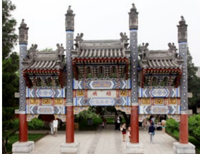
Figure 56: Image reference of memorial arch
